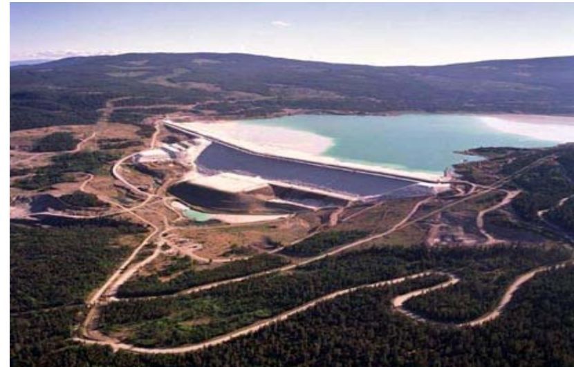
The L-L embankment of the Valley impoundment The Highland Valley Copper Mine is located just outside the town of Kamloops in British Columbia, Canada. The mine produces copper (435,000 tones in 2003) and molybdenum (6405 tones in 2003) concentrates. The tailings pumped to the Valley Impoundment in 2003 were 48.5 million tons.
