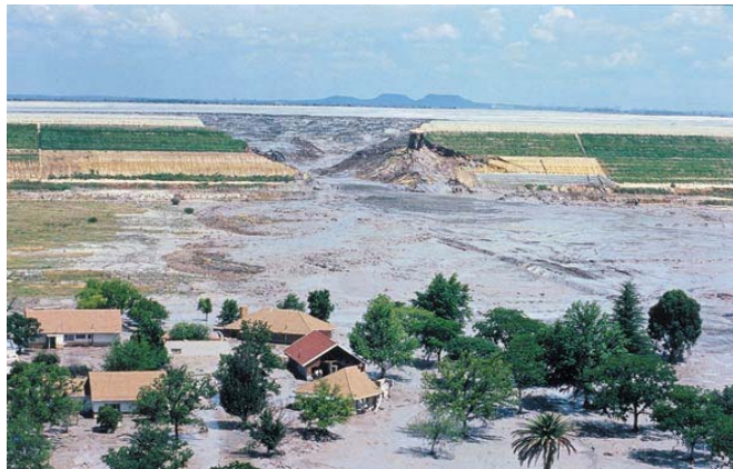
Marriespruit South Africa 1994 Wet tailings
