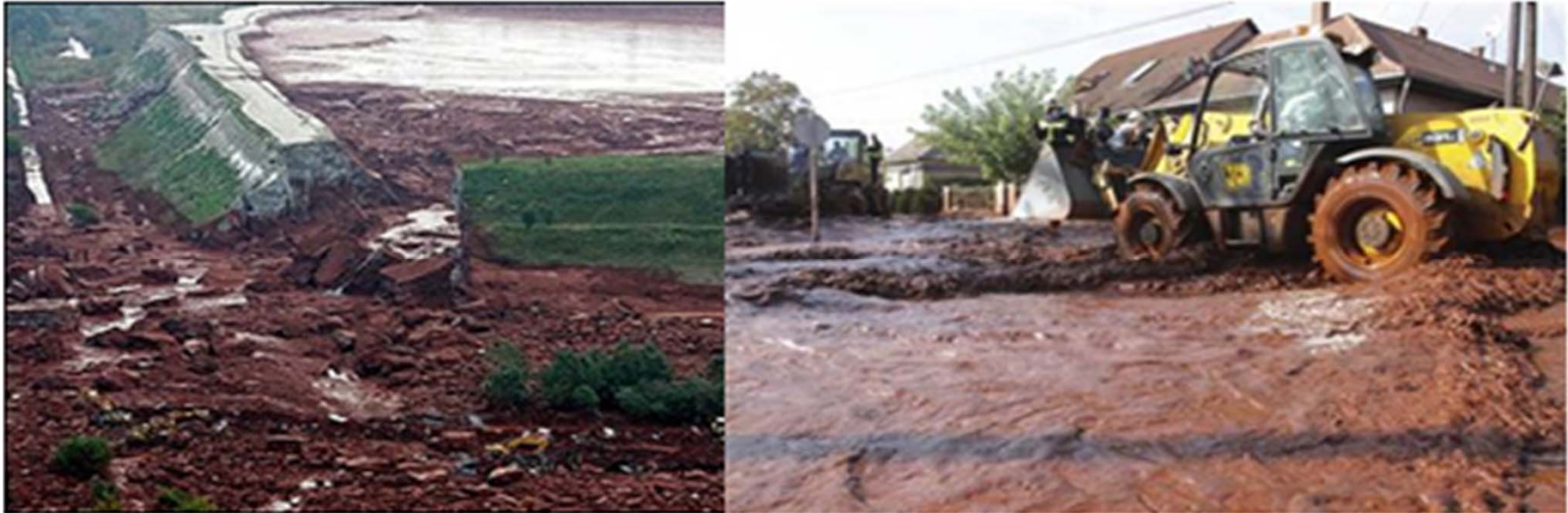
The Ajka Timfoldgyar Alumina Plant Tailings Dam Accident October 4th 2010 in Hungary. Hungary's government estimated that it would cost more than US$51 million and take at least a year to clean up the damage. Hungarian state news service MTI estimated at the time of the accident that Hungary stores about 50 million tons of the red tailings with about 800,000 tons generated annually.
